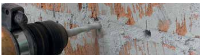
Drilling the holes
