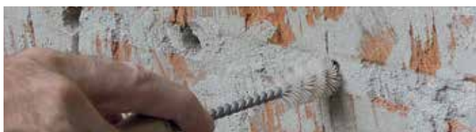
Removing dust & debris from after drilling
