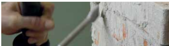
Removal of render from damaged areas
