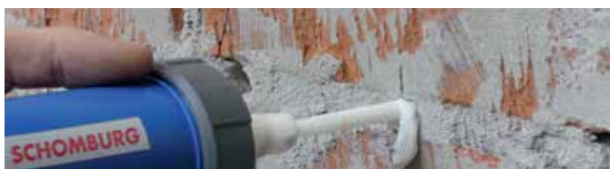
Injecting the cream-consistency AQUAFIN®-i380
