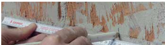
Marking out the bore hole spacing
