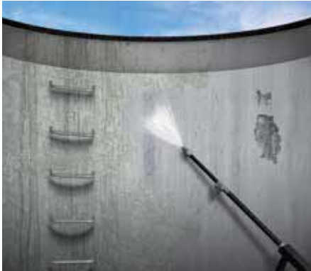
1 Cleaning prior to renovation
