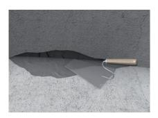
1. Level out damaged areas Repair small crack damage and voids with a trowel or float. Application of ASOCRET-BIS-5/40 "while still wet" onto ASOCRET-KS/HB adhesive slurry.
