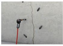
5. Permanently waterproof cracks During application of AQUAFIN-P1, additional injection using AQUAFIN-P4 elastic crack waterproofing is necessary.
