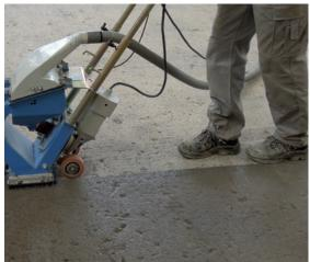
The waterproofing materials must harmonise with the substrate and require the best possible bonding for secure and long-lasting sealing function. For this reason, substrate preparation and its specific requirements are regulated in parts 1 and 3 of DIN 18533. The standard specifies the basic principles and details like the evenness, burr removal, and cleaning, as they apply to every user or installer.
