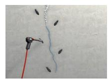
Insert corresponding injection packer into the drilled holes. Press AQUAFIN-P1 into water-conducting cracks. The material reacts with the water to produce a waterproof, tough elastic foam to stop water penetration. The excess foam is removed after curing so it is flush with the surface.
