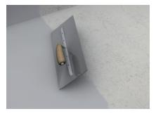
3. Level the surface Apply ASOCRET-BIS-1/6 onto the prepared substrate in the desired layer thickness up to 6 mm in a single application step and processed retroactively using a felt or sponge board.
