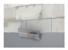
1. Levelling and pre-sealing Levelling of the exposed, load-bearing wall surfaces and application of the pre-seal in one application step with ASOCRET-M30 as a levelling and waterproof plaster. Treat the wall surfaces with ESCO-Fluat beforehand.
