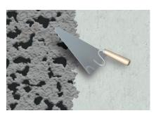
5. Apply restoration plaster Apply up to max. 3 cm THERMOPAL-ULTRA in one application step. After sufficient standing time, the surface may be grid floated or rubbed down.
