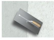
6. Apply fine plaster Apply THERMOPAL-FS33 cementitious fine plaster using trowel techniques in the required layer thickness up to max. 3 mm. After drying, treat the surface with a sponge rubber or a felt or sponge board.
