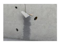
4. Dam up cracks In case of cracks that do not conduct water, the crack area is insulated using ASODUR-EKF. AQUAFIN-P4 is injected after the insulating material cures completely.
