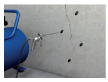
2. Cleaning Clear any drilling debris that has resulted in the drilled holes using oil-free compressed air.
