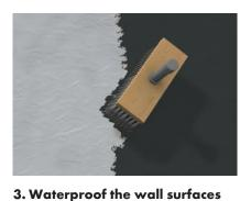
(subject to cracking) After curing the surfaces, AQUAFIN-RB400 is applied in two application steps using a brush/trowel or spray techniques.
