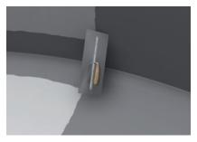
6. Waterproof surfaces Apply AQUAFIN-2K/M-PLUS in at least two application steps using spray, brush, or trowel techniques.
