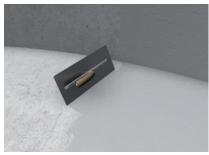
2. Level the surface Apply ASOCRET-BIS-1/6 onto the prepared substrate in the desired layer thickness up to 6 mm in a single application step. The surface may not be processed retroactively with a wide brush or a wet flat trowel. For smooth transitions of the repair surfaces, rubbing with a sponge is possible.
