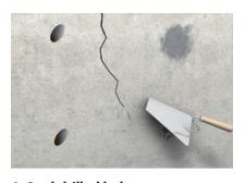
6. Seal drilled holes After the injection resin has hardened, insulation may be removed for visual reasons as required. Seal the drilled holes with ASOCRET-BIS-1/6.
