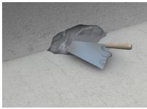
2. Level out damaged areas Close damaged areas and voids with ASOCRET-BIS-5/40 using trowel techniques. Application is completed "while still wet" onto the ASOCRET-KS/HB adhesive slurry.
