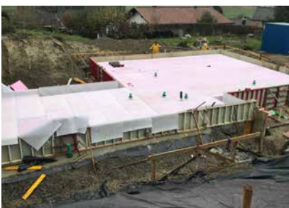
Laid floor slab before the reinforcement was installed
