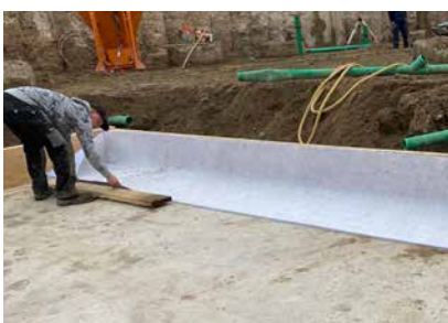
Fixing with a wooden strip
