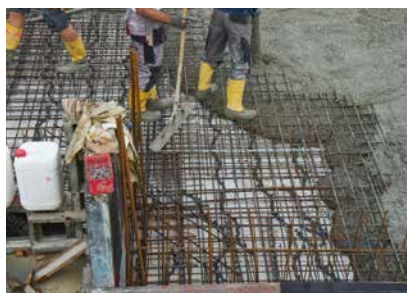
Floor slab after installing the reinforcement
