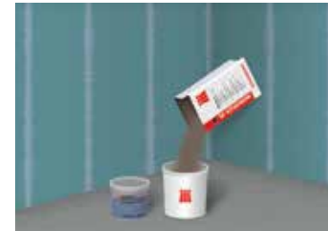
3 Adding the adhesive to a clean mixing bucket
