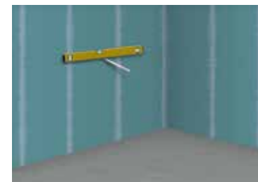
5 Setting out the wall
