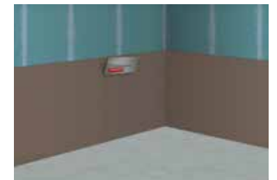
6 Combing out the adhesive bed
