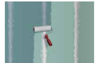
2 Priming the substrate, e.g. with ASO®-Unigrund
