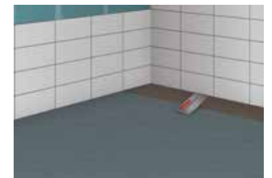
10 Combing out the adhesive bed
