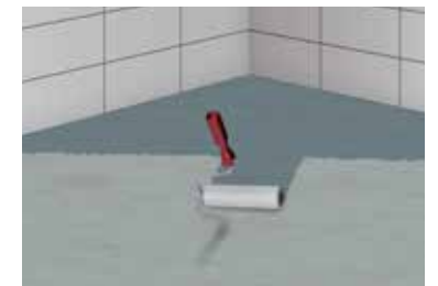
8 Priming the substrate, e.g. with ASO®-Unigrund
