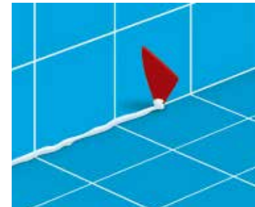
5 Striking off excess silicone sealant
