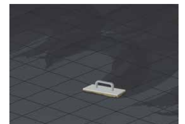
8 Rinsing off surfaces diagonally to the joint direction
