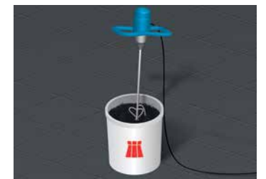
4 Mix the joint mortar
