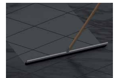
6 Sliding diagonally across excess joint mortar
