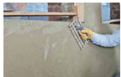
6. Rubbing with a grid float
