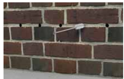
3. Cleaning drill holes
