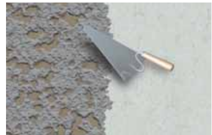
1. Possible backing coat application
