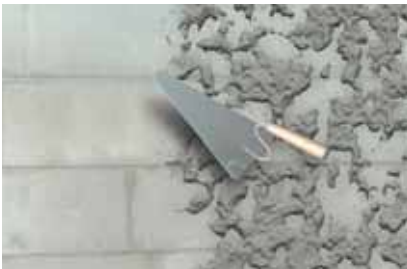
Splatterdash coat/bonding coat
