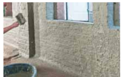
3. Splatterdash coat
