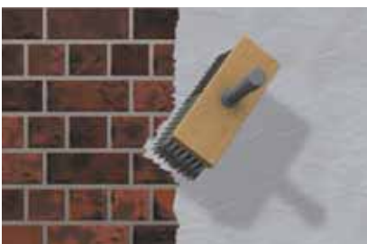
1. Levelling wall areas
