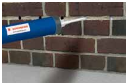
5. Producing horizontal barriers (paste)
