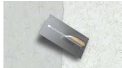
2. Restoration plaster application
