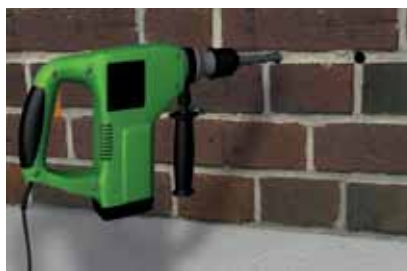
2. Establishing drill holes
