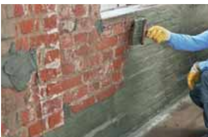
1. Preparation of the wall/floor junction
