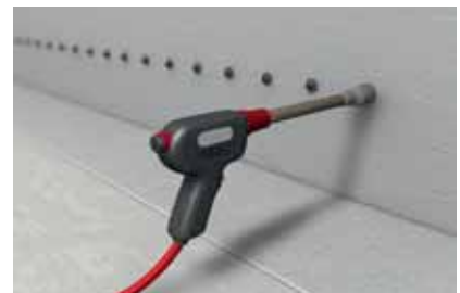
5. Producing horizontal barriers (aqueous)
