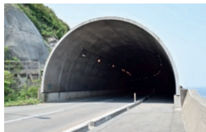
Tunnels and concrete pipes
