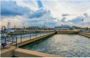
Collection and retaining basins
