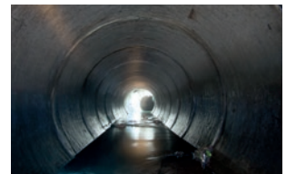
Drain and manhole access points
