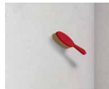
7 Cleaning an absorbent substrate
