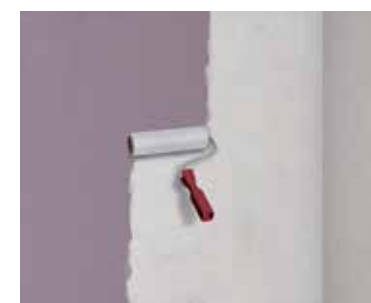
9 Priming the substrate with undiluted ASO®-Unigrund-S
