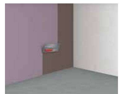
10 Combing out e.g. a thin-bed adhesive
