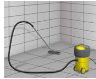
1 Cleaning the substrate
