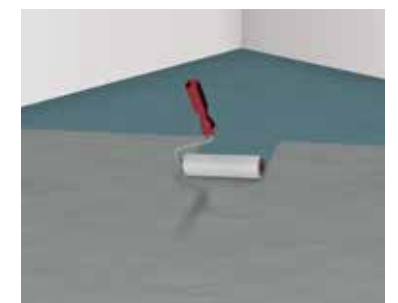
8 Priming the floor substrate
