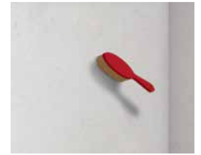
2 Cleaning the wall substrate
