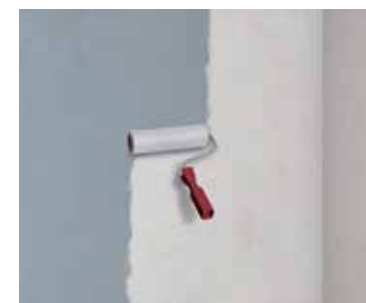
7 Priming the wall substrate
