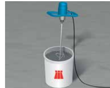
5 Mixing the smoothing compound
