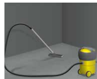
7 Cleaning the floor substrate
