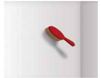
2 Cleaning the wall substrate
