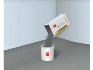
4 Adding the smoothing compound to the pre-weighed water
