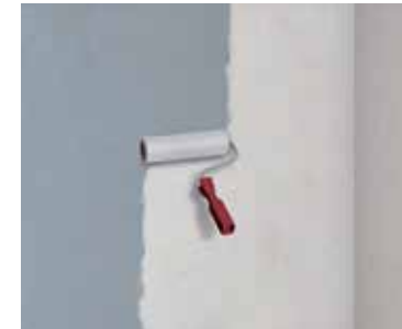
3 Priming the substrate, e.g. with ASODUR®-GBM
