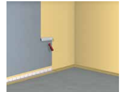
6 Application of the first coat of waterproofing membrane
