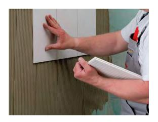
Gypsum fibre board is only permitted as a substrate for moderately exposed wall surfaces in rooms, such as domestic bathrooms. The building board must be protected against moisture damage with a bonded tiled waterproofing.
