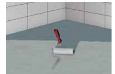
8 Priming the substrate, e.g. with ASO®-Unigrund
