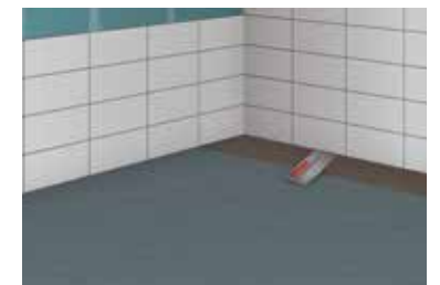
10 Combing out the adhesive bed
