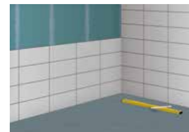
9 Setting out the floor
