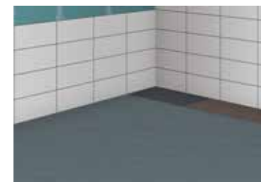
12 Laying the floor tiles
