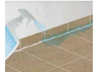
4 Application of a suitable smoothing agent
