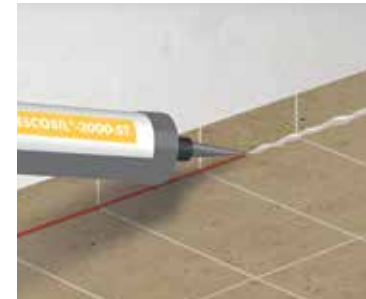
3 Application of ESCOSIL®-2000-ST
