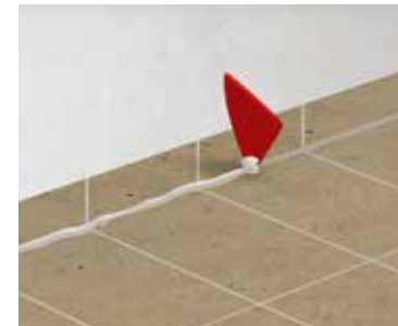
5 Striking off excess silicone sealant
