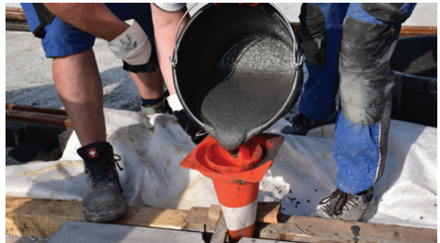
Practical example Grouting concrete elements
