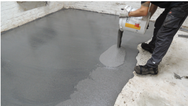
Practical example Application of a flowable levelling layer on concrete
