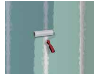
2 Priming the wall substrate
