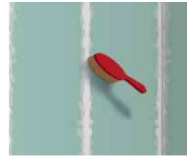
1 Cleaning the wall substrate
