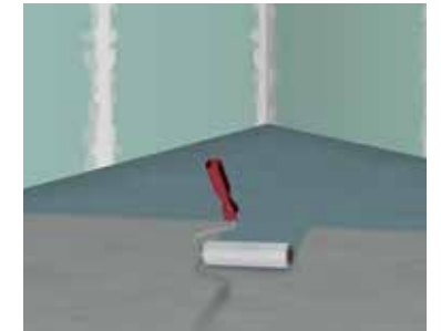
4 Priming the floor substrate
