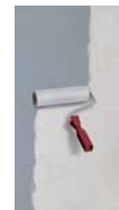
3 Priming the substrate, e.g. with ASO®-Unigrund
