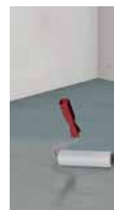
3 Priming the substrate, e.g. with ASO®-Unigrund
