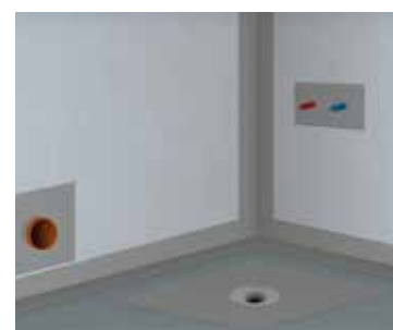
9 Overcoating the ASO®-Joint-Tape technology and waterproofing the surface with a suitable SCHOMBURG bonded waterproof coating
