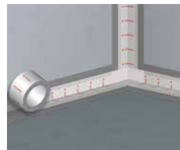
5 Bonding ASO®-Joint-Tape-2000 in the first coat of the waterproof membrane
