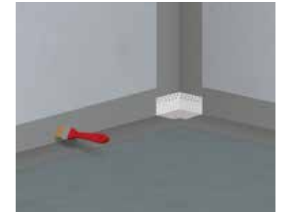
4 Bonding ASO®-Joint-Tape-2000-S-Corners in the first coat of the waterproof membrane
