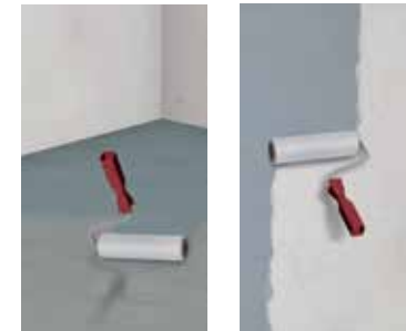
3 Priming the substrate, e.g. with ASO®-Unigrund
