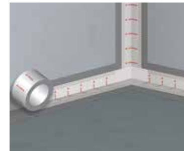
5 Bonding ASO®-Joint-Tape-2000-S in the first coat of the waterproof membrane
