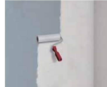
3 Priming the substrate, e.g. with ASO®-Unigrund
