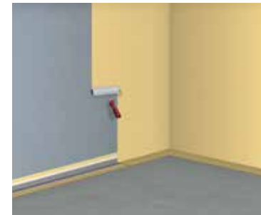
5 Application of the first coat of waterproofing membrane
