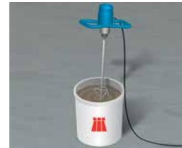
5 Mixing the waterproofing membrane
