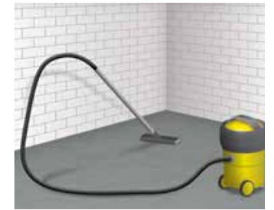
2 Cleaning the substrate
