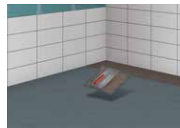
11 Applying a contact layer with large format tiles
