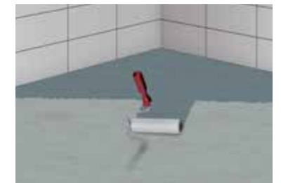
8 Priming the substrate, e.g. with ASO®-Unigrund
