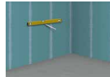
5 Setting out the wall
