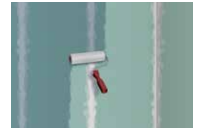
2 Priming the substrate, e.g. with ASO®-Unigrund
