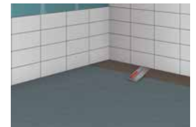
10 Combing out the adhesive bed
