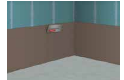
6 Combing out the adhesive bed
