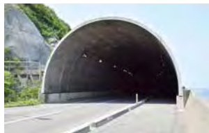
Tunnels and concrete pipes
