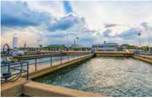
Collecting and retaining basins
