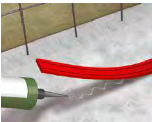
1. Bonding using a mounting adhesive
