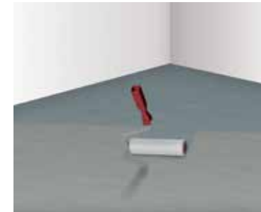
3 Priming the substrate, e.g. with ASO®-Unigrund
