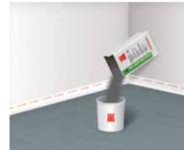
5 Adding the levelling compound to the pre-weighed water
