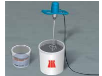
6 Mixing the levelling compound
