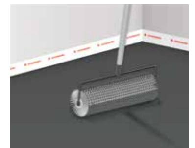
8 Evening and de-aerating the fresh levelling compound
