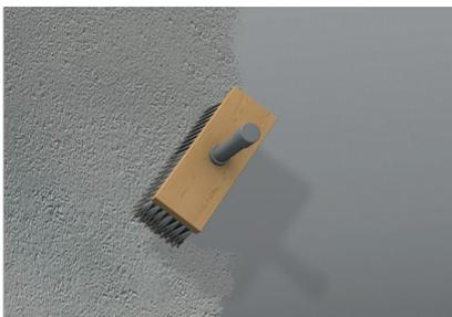
**7. Application of AQUAFIN®-IC** Dampen all surfaces to be waterproofed with clean water. Apply two layers of AQUAFIN®-IC in the required useful quantity with a roofer's brush, wide brush, or using spray techniques. Apply the second layer while the first layer is still sticky and has not yet dried out.
