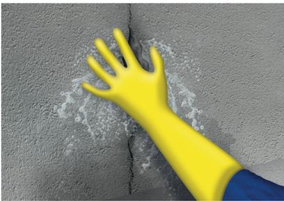
**4. Plugging the water ingress points** Press the formed plug into the leak position. Hold the plug firmly in place by hand until it has hardened. Process the plugged position immediately afterwards with a trowel.
