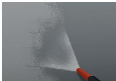
**8. Retreating existing surfaces** The fresh coating must be protected against weathering influences, e.g. sunlight, wind, rain, and frost, etc. The waterproofing layer must be kept damp for at least 3! Complete the first damping after approx. one day.
