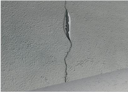
**1. Open cracks and damaged areas** Remove all loose components from the cracked and damaged areas. Break open the static cracks up to a width of at least 20 mm and a depth of at least 25 mm.
