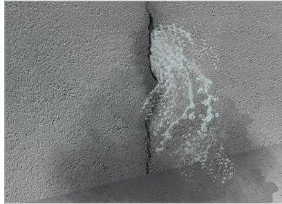
**2. Immediate waterproofing for water breakthroughs** Water breakthroughs are sealed professionally with rapidly hardening cementitious FIX 20-T sealing mortar.
