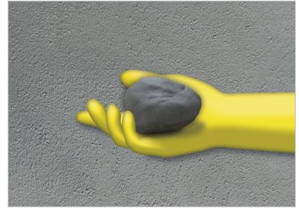
**3. Mix the FIX 20-T** Mix a powder quantity corresponding with the water breakthrough together with approx. 25% water to produce a homogenous consistency able to be kneaded. Form a suitable plug by hand. Work quickly: The pot life is only approx. 3 minutes!
