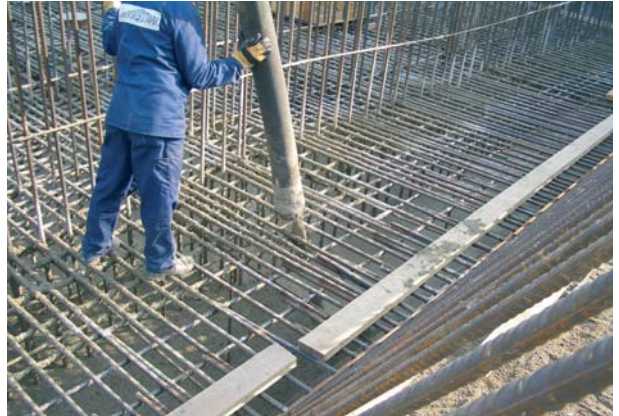
10 tonnes BETOCRETE 406 (FM) during application: Construction site in Kosice, Slovakia.
