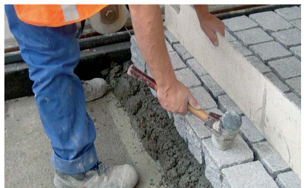
Laying the pavers in INDUCRET®-VK-Bettungskleber.
