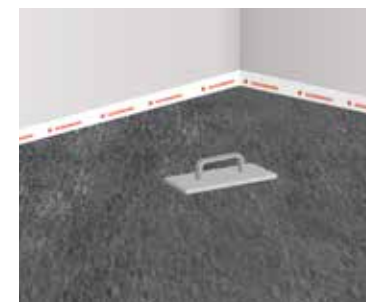
7 Rubbing up and finishing the screed surface
