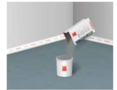
2 Filling the clean mixing bucket with screed mortar
